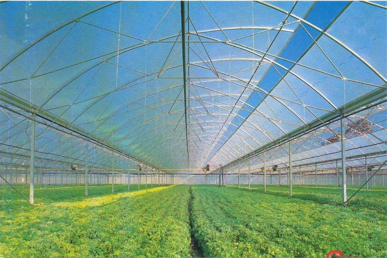
**Folienblock 9m 60 SR. Dachlüftung 35 %.**
