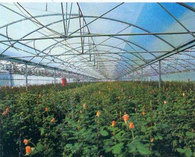
**Folienblock 8m SR. Dachlüftung 50 %.**
