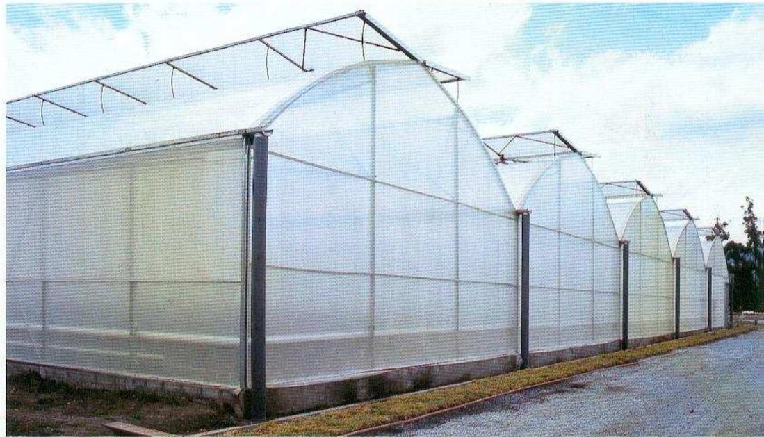
**Folienblock 9m 60 SR. Dachlüftung 2 x 20 %.**
